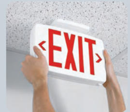
3. Attach housing to butterfly bracket and connect input leads.
