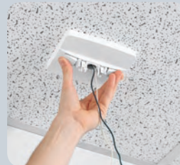
2. Attach canopy to butterfly bracket. No fasteners needed.
