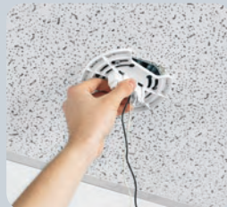
1. Connect leads and twist butterfly bracket into place using existing J-box screws.
